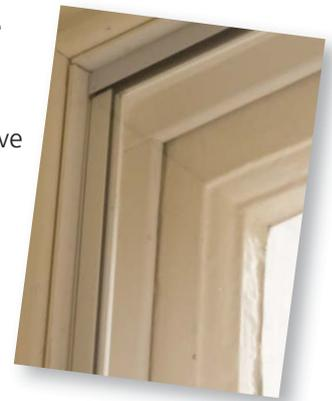
Sash windows are notorious for letting in cold air. You can get clear, light-weight acrylic panels to fit over the glazed frames, but these don't cover the many gaps on the sides, top and bottom that make sash frames particularly draughty.
