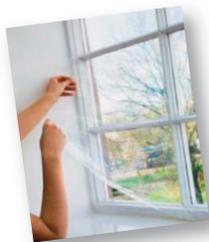
Enough film to cover a large bay-window costs £10-15 and is available from DIY stores. The film is simple to remove, though it can damage paintwork.
