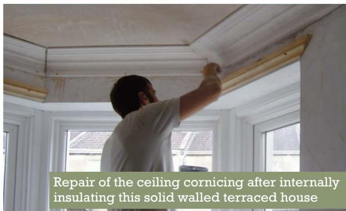
Repair of the ceiling cornice after internally insulating this solid walled terraced house
